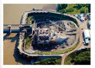
an average annual output of approximately 239 million kilowatt-hours (kWh), enough to power approximately 22,000 homes. The site will include an intake approach channel, a reinforced concrete powerhouse and a tailrace channel. The powerhouse will feature two horizontal FERC rated 17.5-MW bulb-type turbine and generating units with an estimated total FERC rated capacity of 35 MS at a gross head of 20 feet. A 1.6-mile 138 kV transmission line is planned to connect to the plant.
